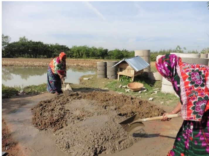
Nargis and Parul mixing concrete
